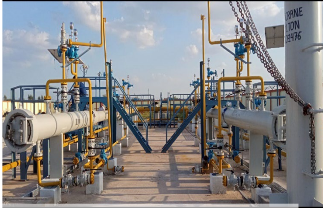
Station Piping Works at Sultanpur-Jhajjar Pipeline Project
