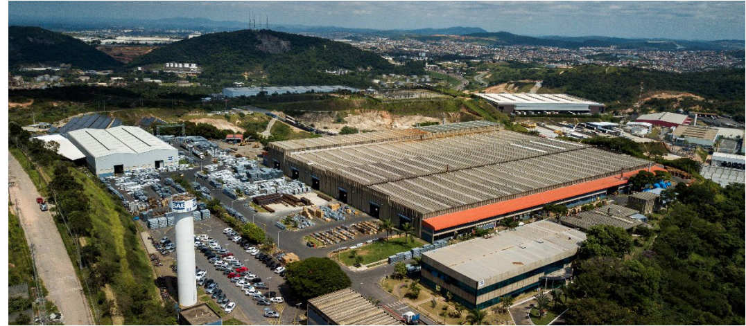
Tower Manufacturing Facility, Brazil
