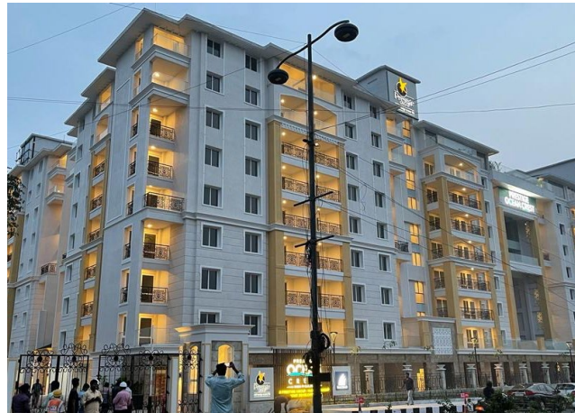
Construction of luxury residential project in Goa
