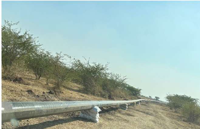
Kandla Gorakhpur Pipeline Project
