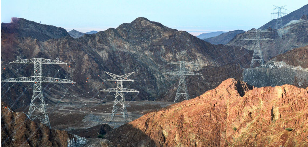
400 kV IBRI-New Rustaq O/H Transmission Line, Oman
