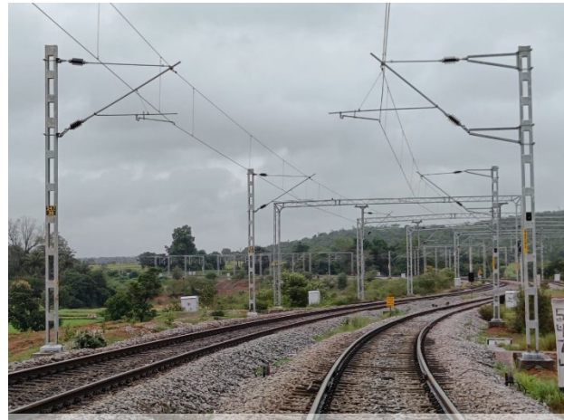
Hubli - Tinaighat Railway Electrification project, Karnataka
